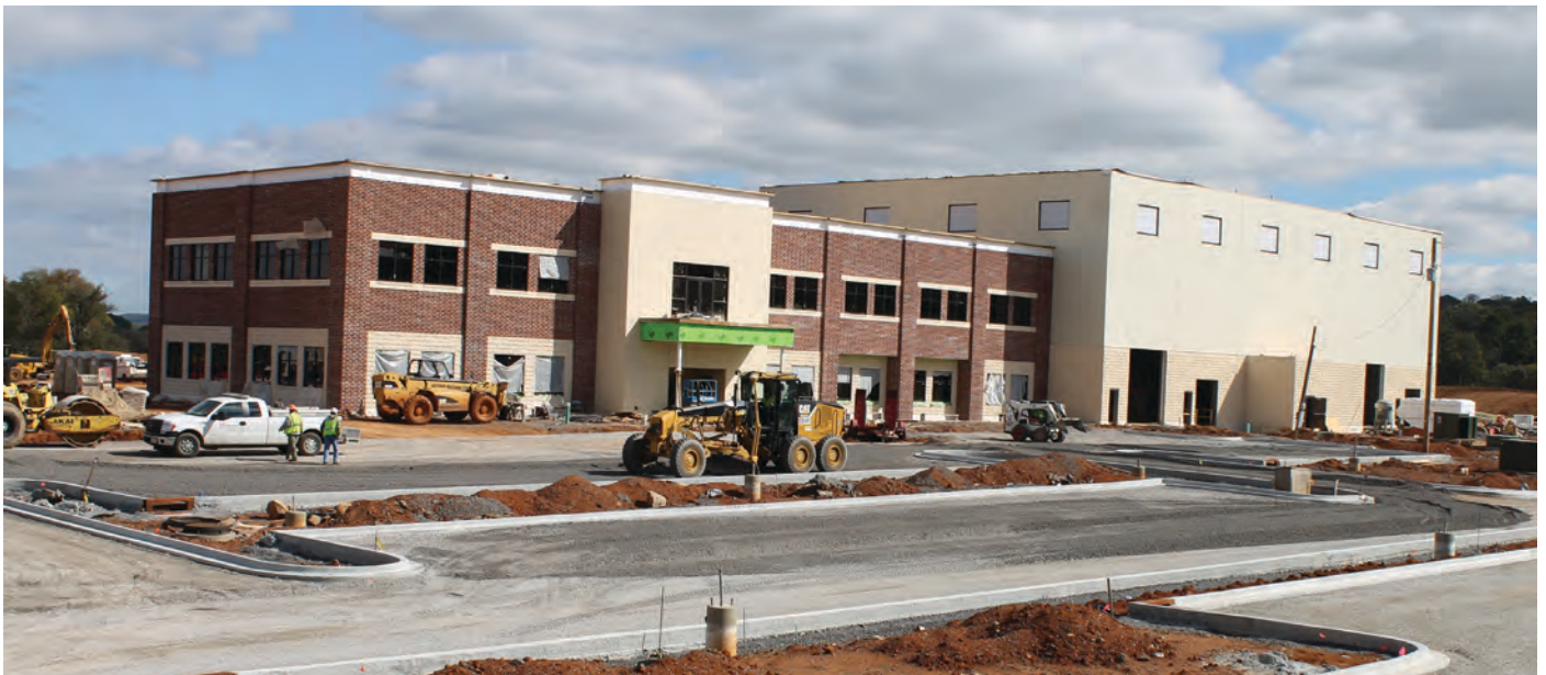
ProNova facility construction continues at Pellissippi Place.
